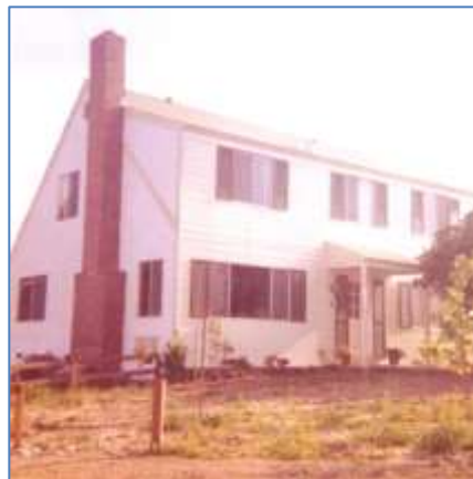
Figure 3-- Chimney and wood box door.
